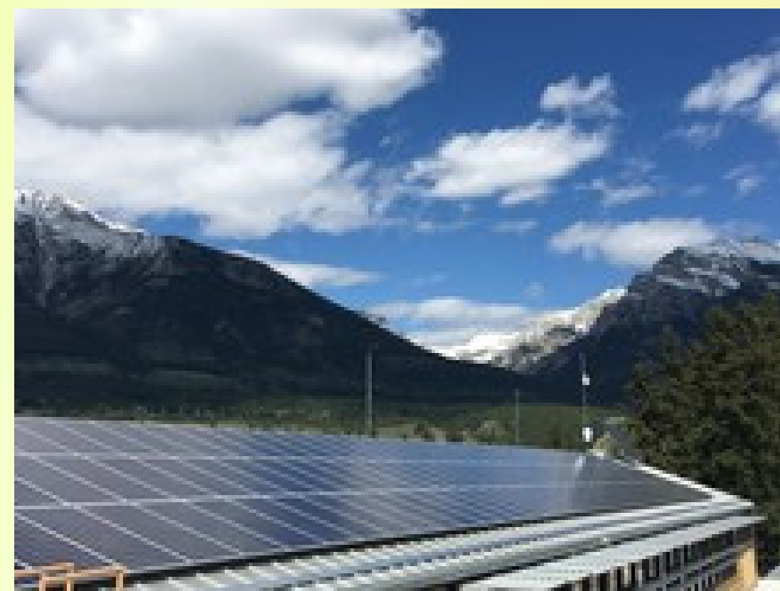
Figure 1: The Town of Canmore, 64.6kW Civic Center Rooftop Solar Array
